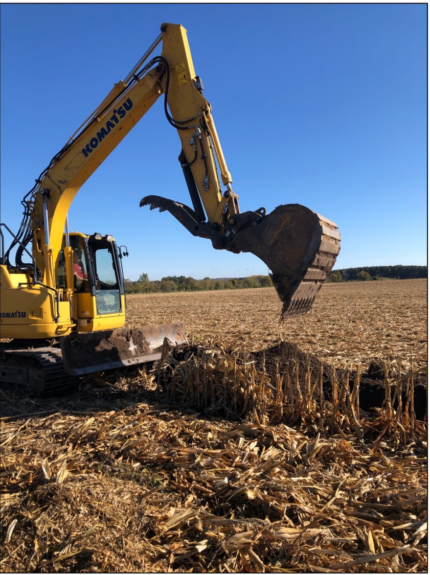
Using an excavator to install wick lysimeters October, 2021
